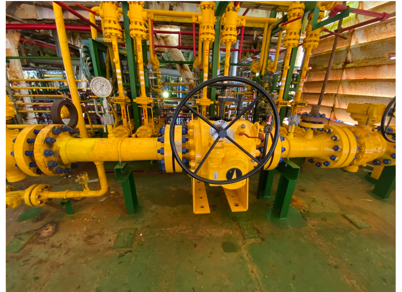
Integrated Pig Ball Valve
